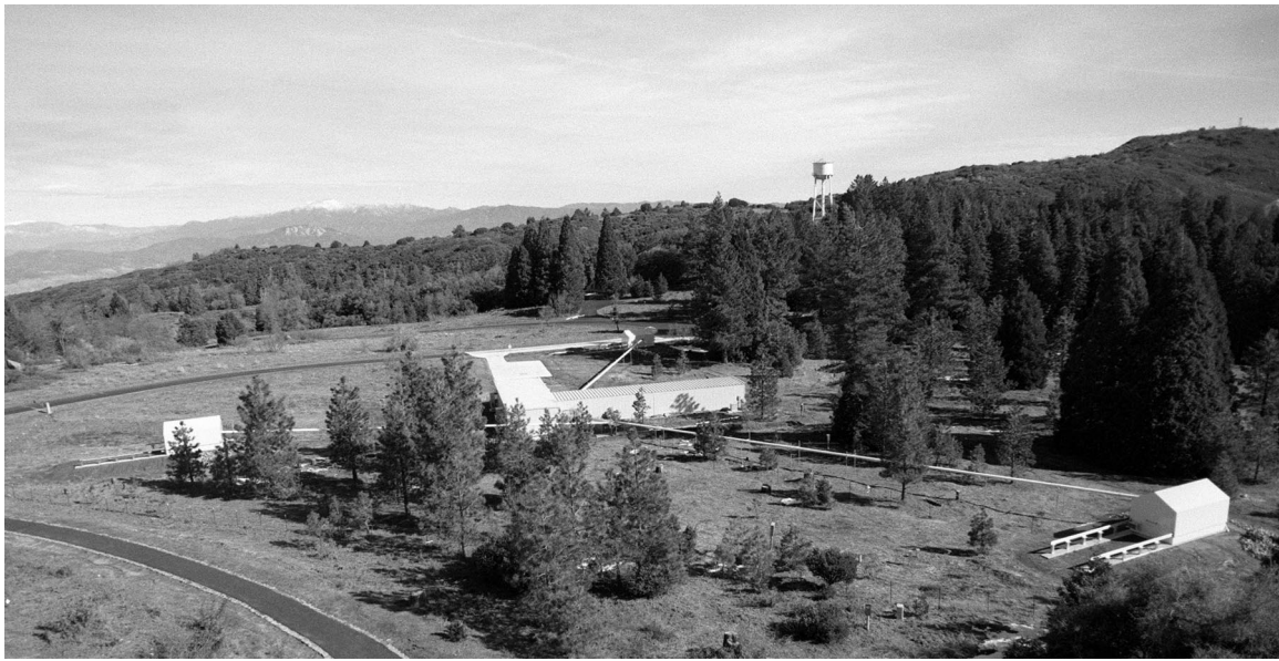
FIG. 1.—Photograph of the Palomar Testbed Interferometer (PTI) at Palomar Observatory taken from the catwalk of the 5 m Hale telescope looking northeast. The driveway and adjacent road are painted white to minimize daytime heating.
