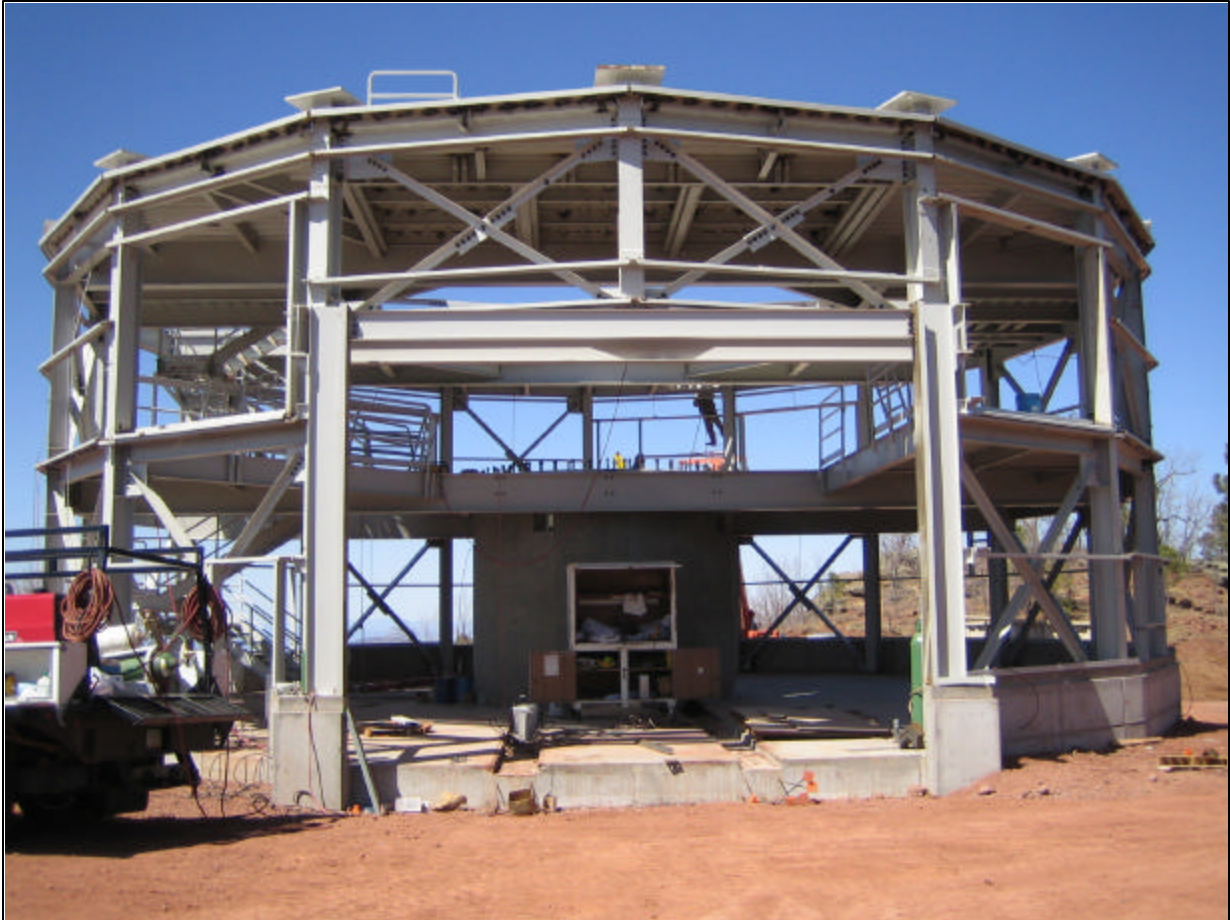
Figure 3-2: DCT Enclosure Construction Progress, April 2006
